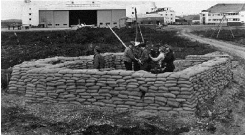
75mm Skysweeper emplacement, Ladd Air Force Base, Fairbanks, AK, 1950s.
