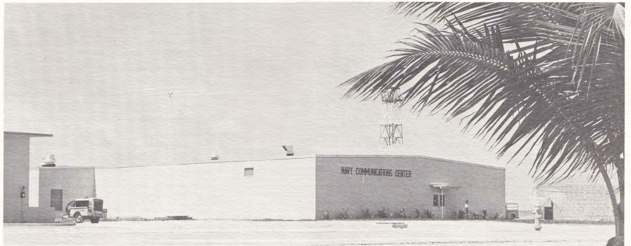
Navy Communications Center — 110' x 82' structure with 8" concrete block walls and structural steel frame. Houses extensive communication facilities and in one shielded room very delicate instruments.
