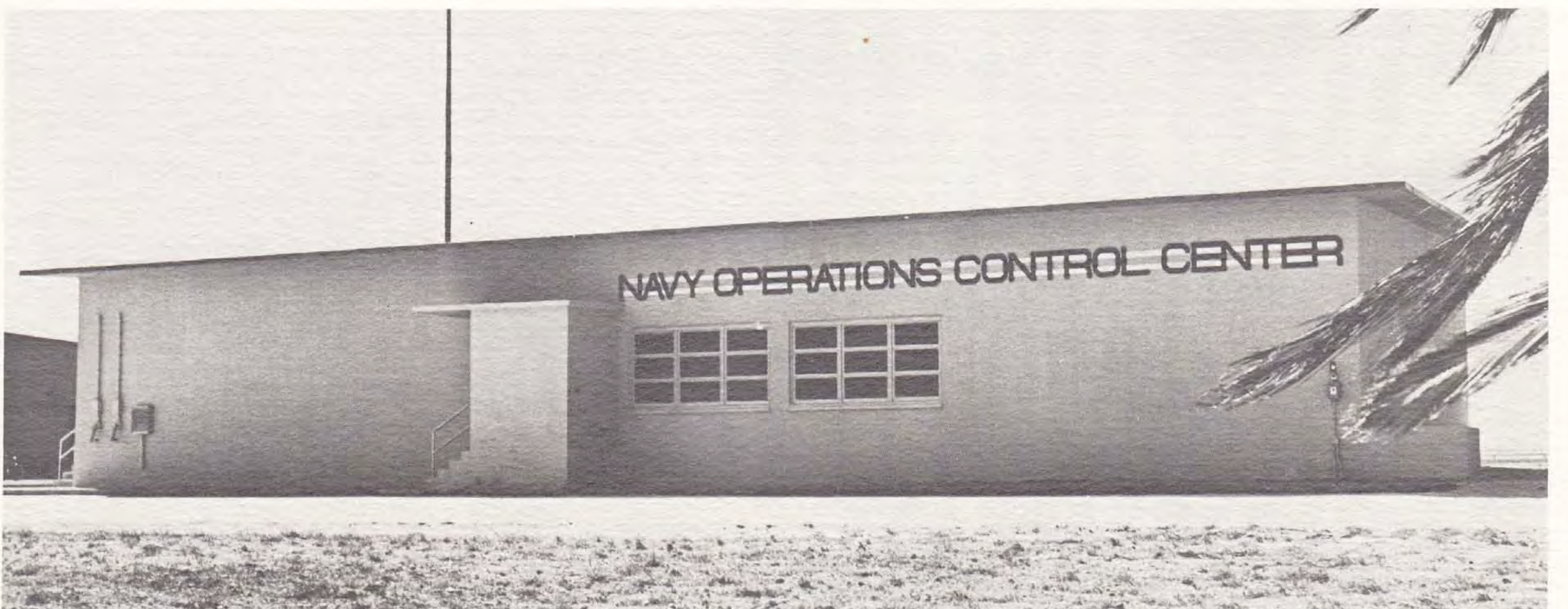
Navy Operations Control Center — 96' x 60' structure with 12" reinforced concrete block walls. Building features 2495 sq. ft. of movable metal floor system on 3' adjustable jacks.
