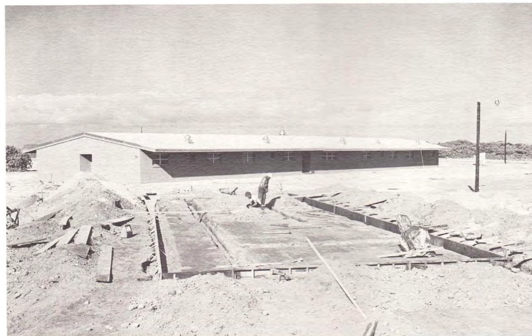
4 Dormitories — Provide accommodations for 144 men. Concrete block, air-conditioned buildings, with 28,500 sq. ft. total floor area. Ancillary building foundations in foreground.
