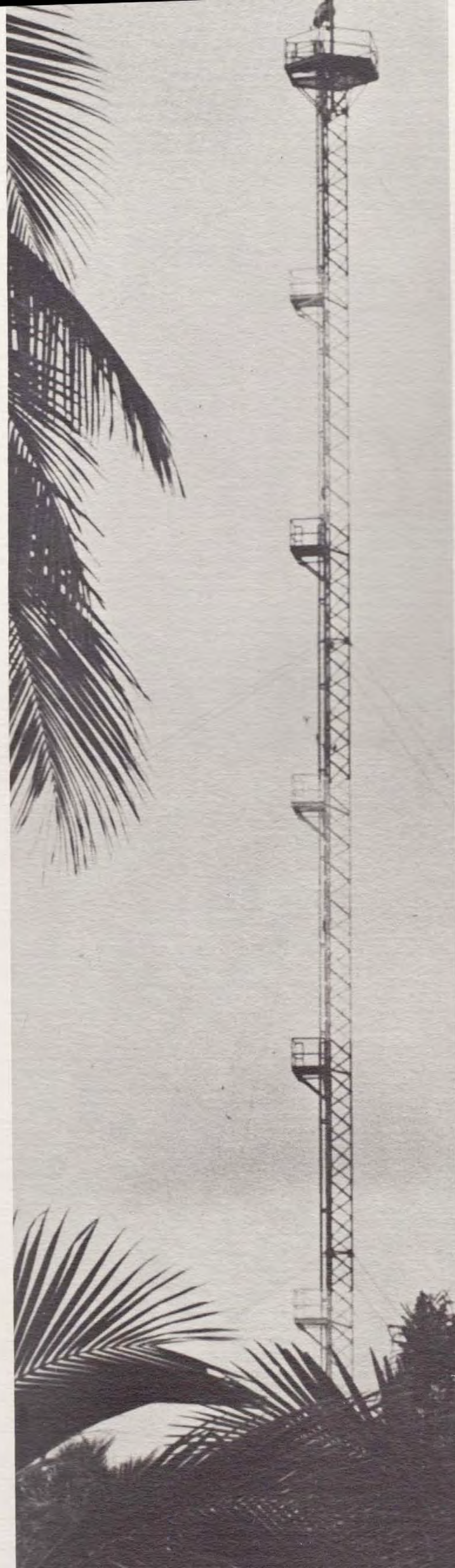
Boresight Tower — 218 ft. high on Roi-Namur. Another tower, 264 ft. high, is located on Ennurgarret Island — 6000 ft. from Tradex Radar Antenna.
