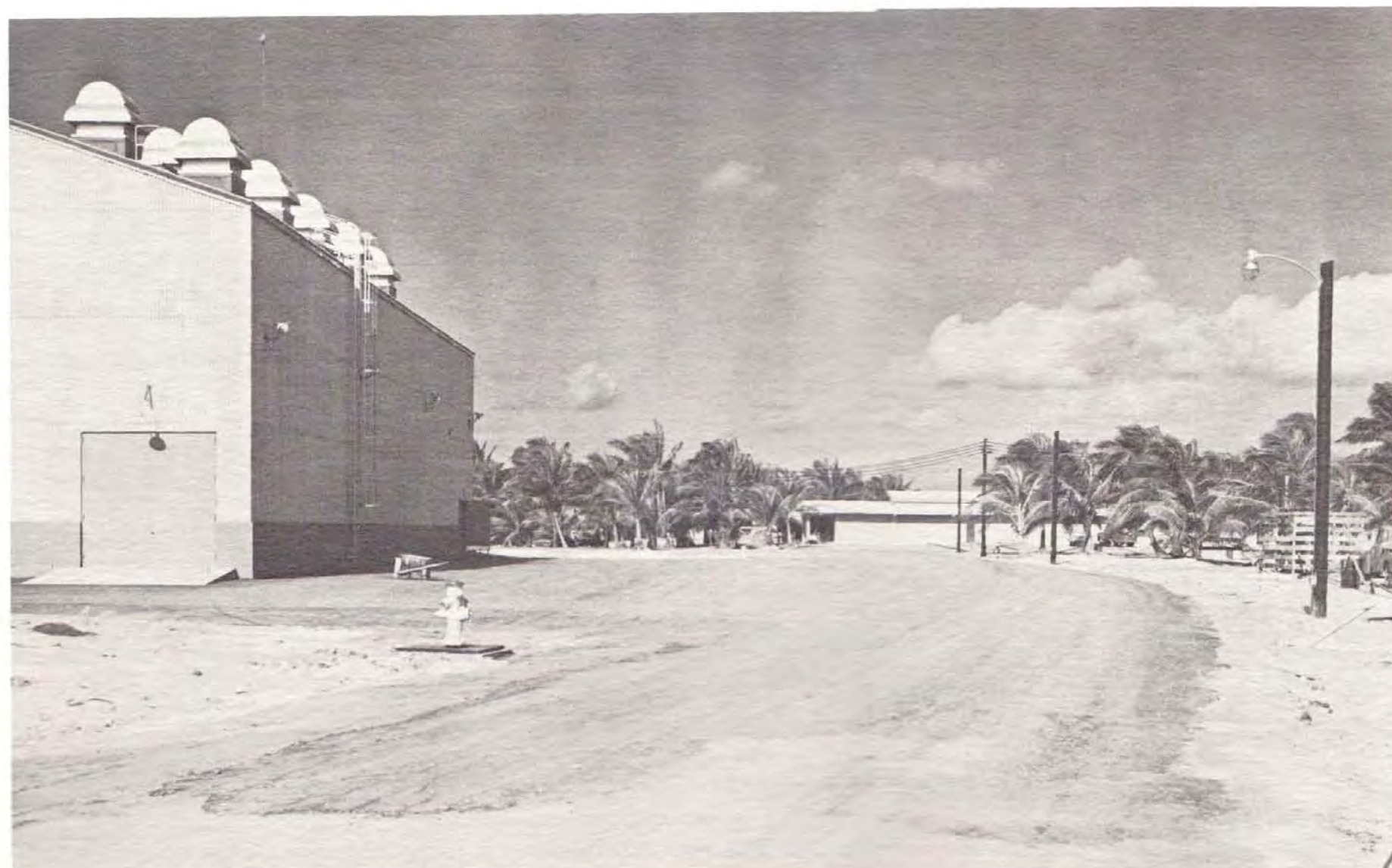
Power Plant at Left — 143' x 58' x 43' high steel framed building, housing seven diesel engine-generator units for precise power. Part of new roadway at right.
