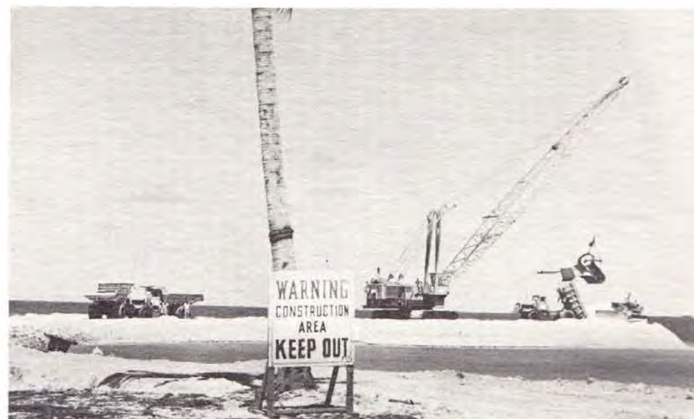
Equipment working on Mobile Homes Park fill. This spread is only a small part of the total Pacific-Martin-Zachry equipment in the Marshalls.
