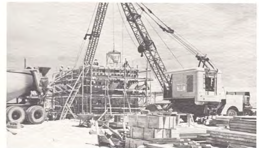
Placing concrete, part of the 69,500 c.y. placed for Nike-Zeus. Another 23,300 c.y. was placed on Roi-Namur.
